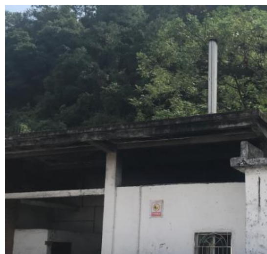
炉灶废气排气筒
